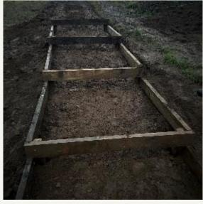
We are also happy to report that the planned extension to the Hilltop Path has now been completed. This work was undertaken to address the particularly muddy and treacherous section at the top of the original path. There have been two new sections of steps added, and a connecting section of path over the previously muddy part. The path now finishes on the hilltop meadow, and we hope this extension will improve access and address safety concerns.
